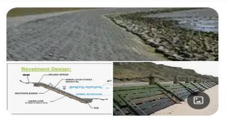
A revetment in stream restoration, river engineering or coastal engineering is a facing of impactresistant material applied to a bank or wall in order to absorb the energy of incoming water and protect it from erosion.
